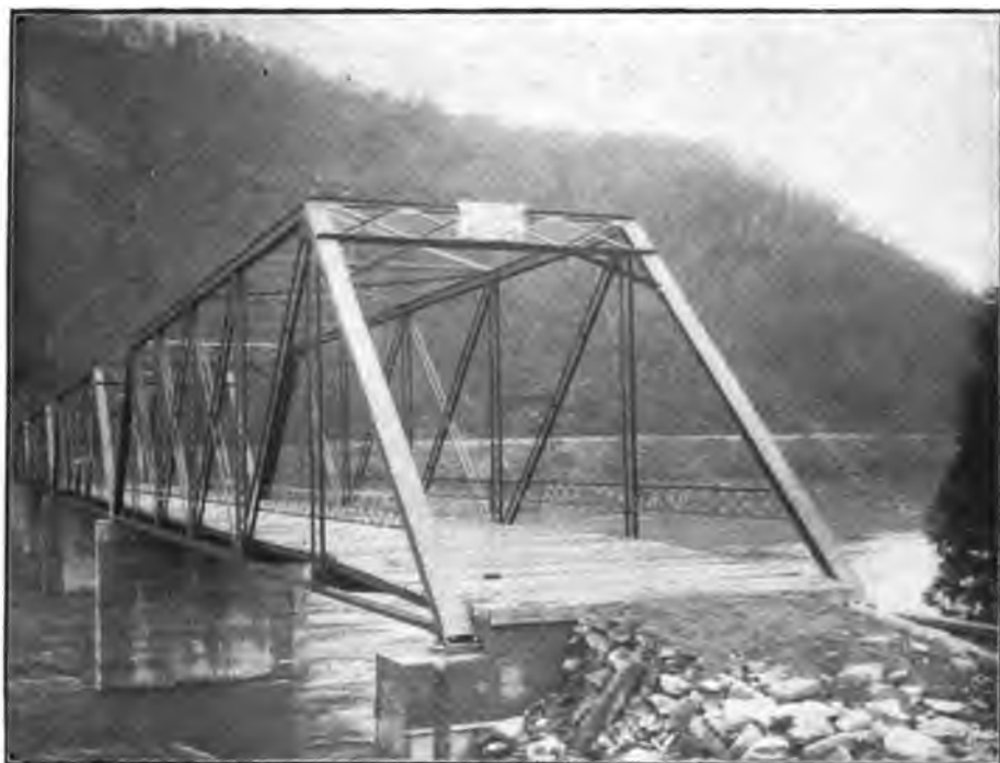
FOSS BRIDGE. Built by Charles Louis Miller, 1907.
